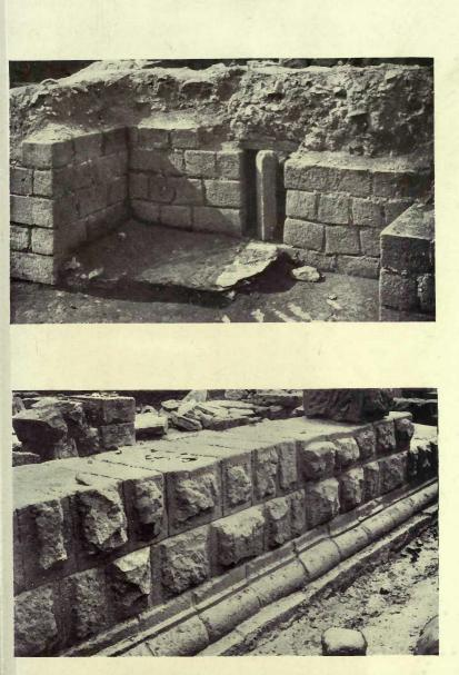
FIGS. 72, 3. WALL OF GRANARY AND 'RUSTICATED' MASONRY WITH MOULDED PLINTH, CORBRIDGE
